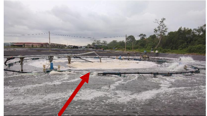
Control Pond : Foam observed heavily at center
